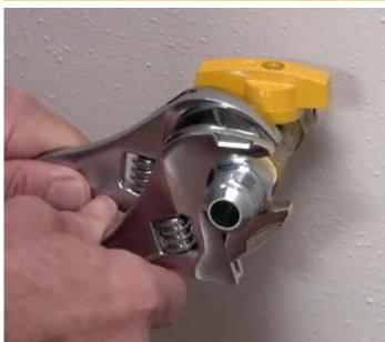
▲ Turn off gas supply before disconnecting old appliance. In absence of manual shut-off valve near appliance location, gas MUST be shut off at main valve, near meter.
